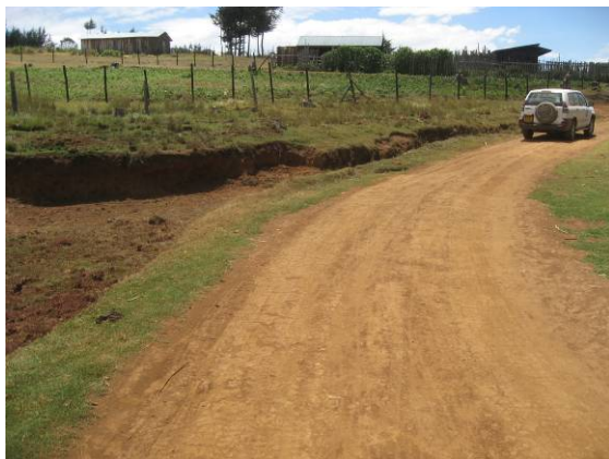
Figure 15. The road situation after two years of maintenance at the same place as in Figure 14 (Kenya)
